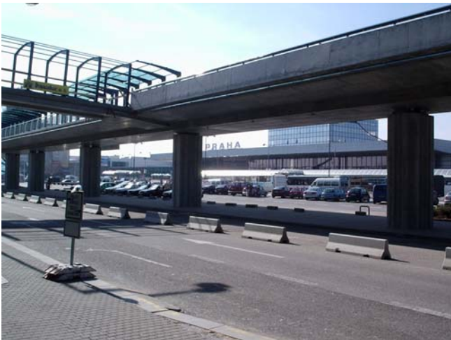
Figure 5 - Scaffold bridge at the Prague airport
